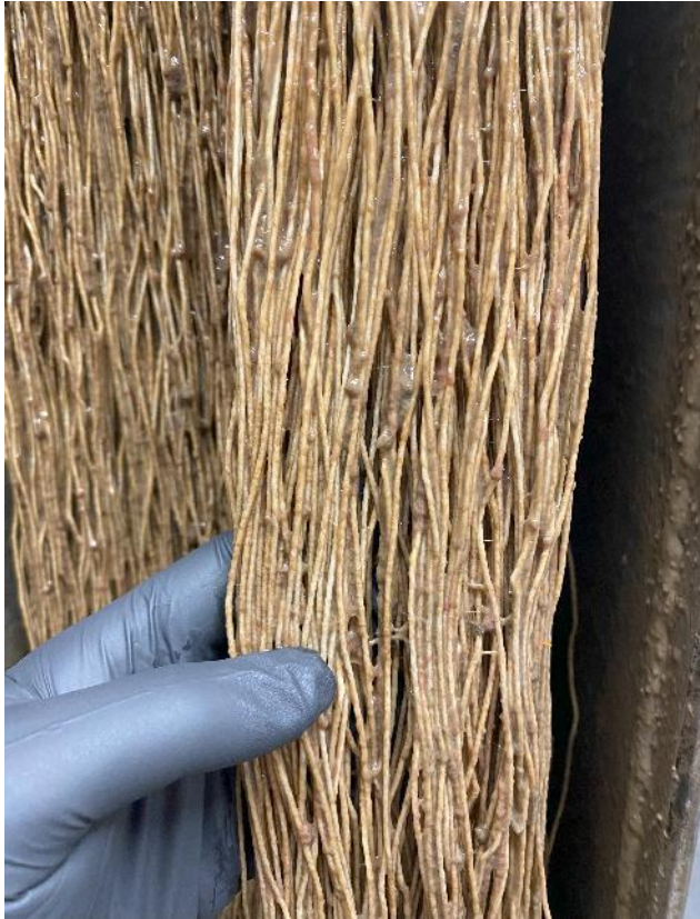
May 15th - Mid Secondary Clarifier Feed
