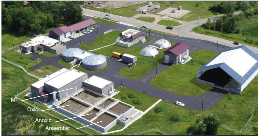
memDENSE installation at Detroit Lakes, MN, USA
