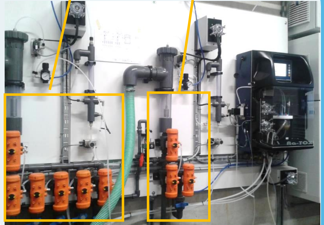
Sampling with EZ9100 external filtration system
