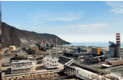
Fujairah 1 Independent Water and Power Plant Fujairah, UAE
