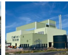
UK 85MW and 130tph steam
