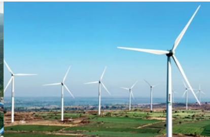
Rojwas wind power assets Madhya Pradesh, India
