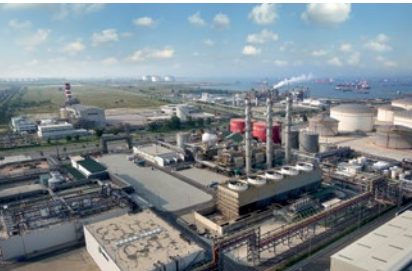
Multi-utilities facilities Jurong Island, Singapore
