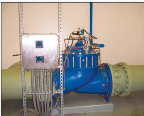
Modulating Level Control with Metering
