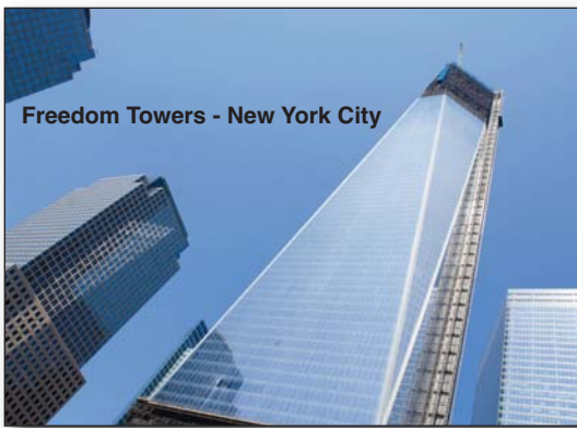
Commercial High-Rise Fire Protection: Breach Control, Pressure Reducing, Pressure Increasing, Fire Pump Control, Pump Check and Air Release
